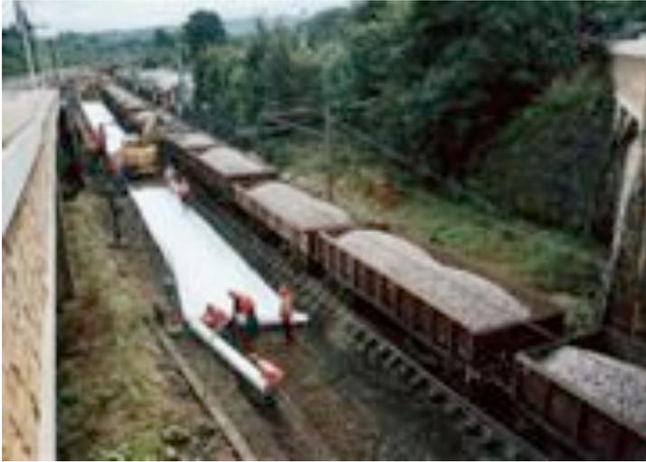
*Engineering work taking place at Crossflatts at end of September, showing the waterspray membrane prior to ballast being laid.
